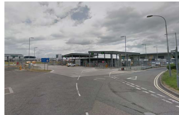
Figure 7. Northwestern Zone - Security Control North
