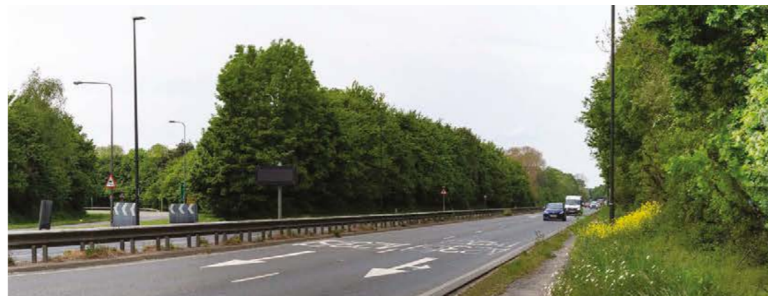
Figure 87. A23 Footway Looking North-West
