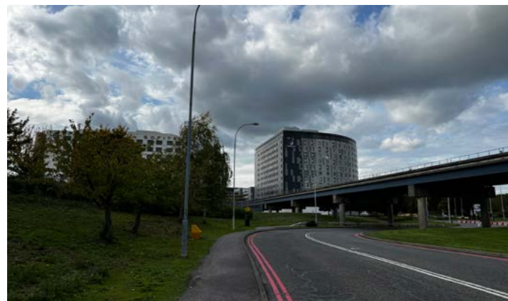
Figure 86. Perimeter Road North view towards NT Hotels
